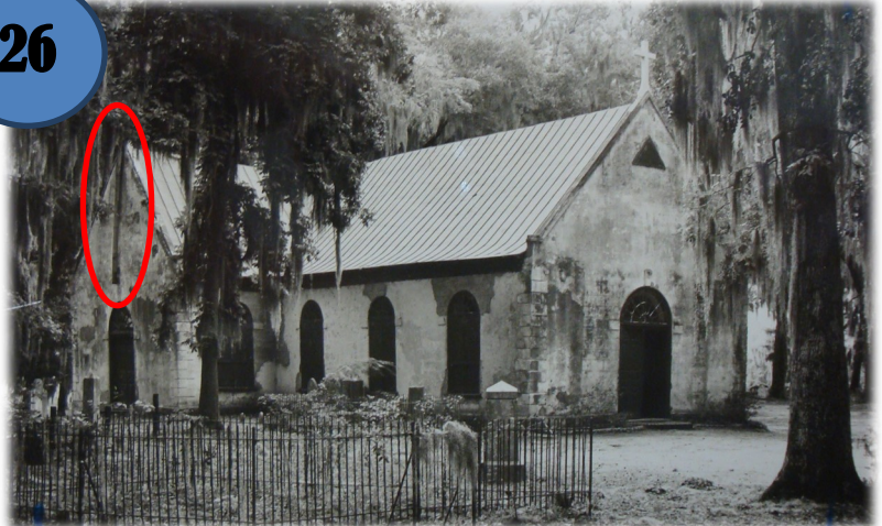
Flue running up the north gable end of the church, Charleston News and Courier , 1957; courtesy of the Evening Post Publishing Co.
