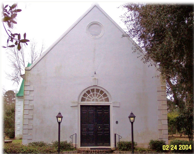
West end of the church, 2004; courtesy of Richard Marks Restorations and Old St. Andrew's.
